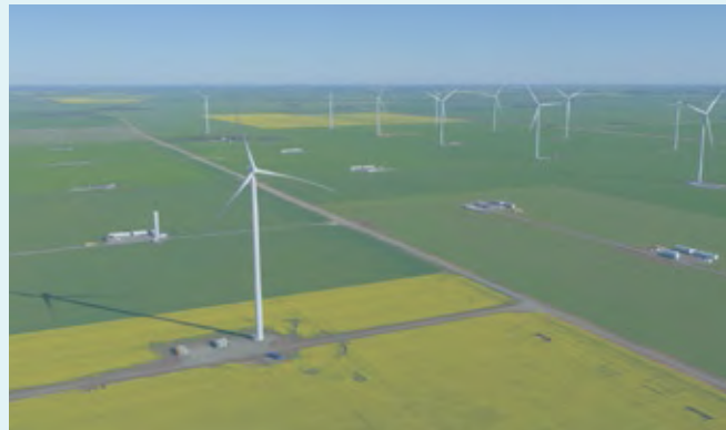
Murra Warra I Wind Farm , Private Infrastructure
